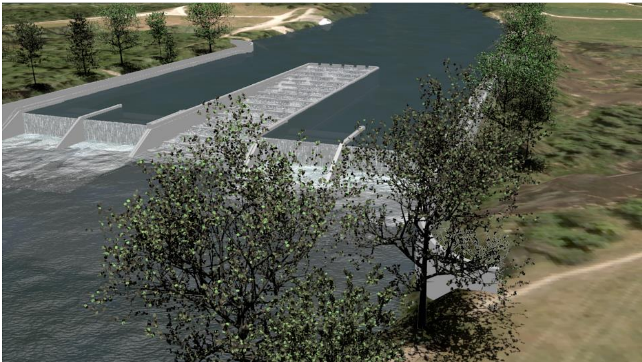
Figure 2: Visualization of the TUM-MSHPP. Eco-migration corridors mainly for upstream migration are positioned in the axis and at the river banks (courtesy J. Frank).
