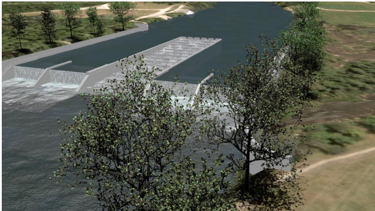
Figure 2: Visualization of the TUM-MSHPP. Eco-migration corridors mainly for upstream migration are positioned in the axis and at the river banks (courtesy J. Frank).
